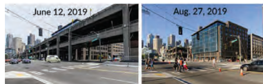
Alaskan Way Viaduct Before and After Source: WSDOT
