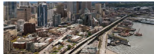
Alaskan Way Viaduct (SR99) Source: WSDOT
